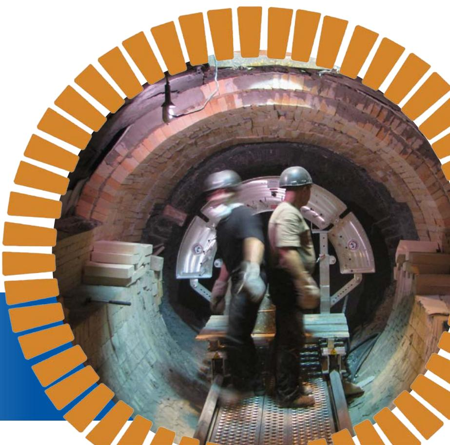
Arch stabilizer post to adjust proper distance of arch from shell.
