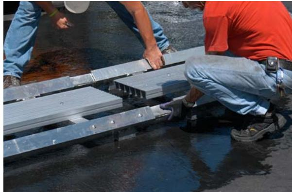
Lightweight mobile trac can be easily assembled and manually moved up kiln as brick work progresses
