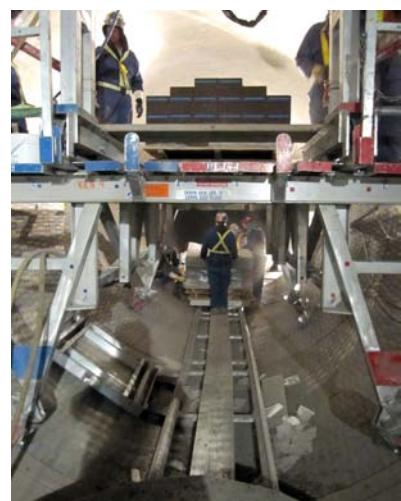
Two men can easily **push a 4,000 lbs pallet** of brick up the kiln. **Multiple transfer carts** with same capacity can run along same trac.
